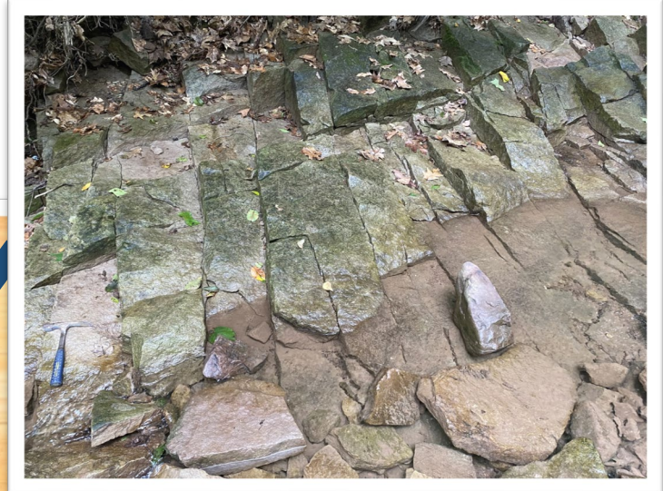
Fractures in Rock At Ground Surface
